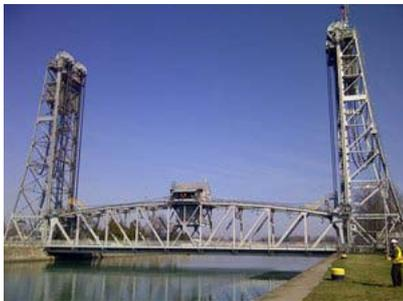
Vertical-lift drawbridges are unique structures. To provide clearance for vessels on waterways, the entire road or rail section is lifted vertically between two towers. Counterweights, equal to the weight of the road section, reduce the amount of mechanical force needed to move the section upward or downward.
